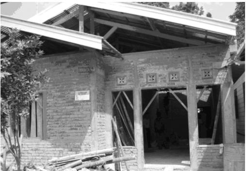
Two common house types suitable for Haiti *Top:* Timber frame with masonry skirt wall *Bottom:* Confined masonry, done well
