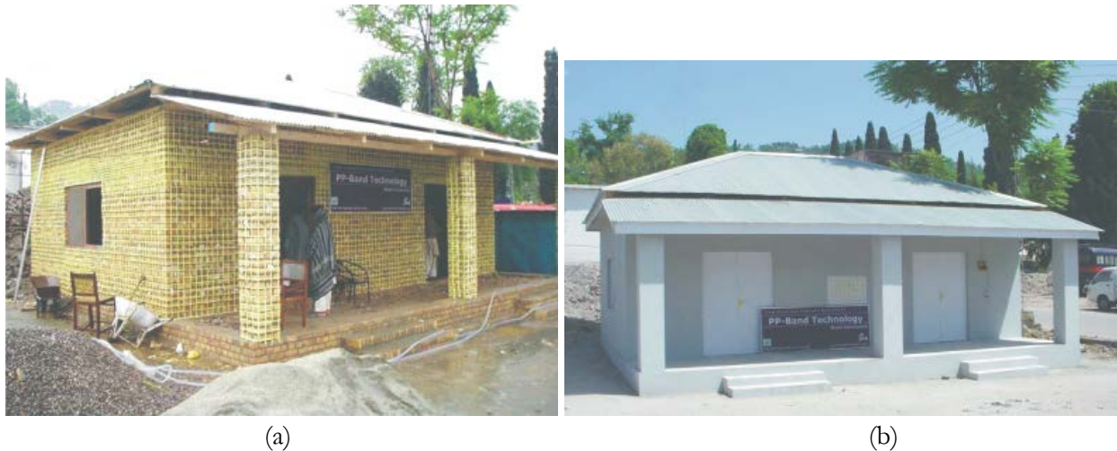
Figure 4. Retrofitted house in Pakistan before and after application of covering mortar layer. Note that the mesh is also applied to the inner face of the walls, with inner and outer meshes connected with through-wall ties. Photograph: Meguro Lab, Tokyo University
