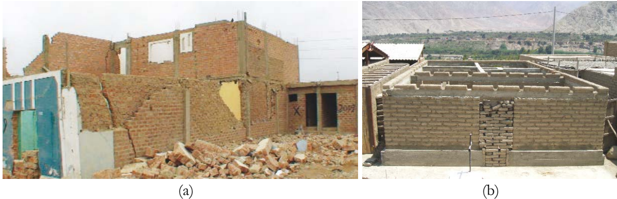
Fig 3. Non-engineered structures using modern construction methods resulting from the negative perception of adobe but limited means of the homeowner: a) Non-engineered confined masonry dwellings in Chíncha that performed badly in the 2007 Peru earthquake b) Non-engineered hybrid structure in Lunahuaná displaying slender adobe walls with long clear spans supporting a heavy concrete ring beam with no vertical tie members
