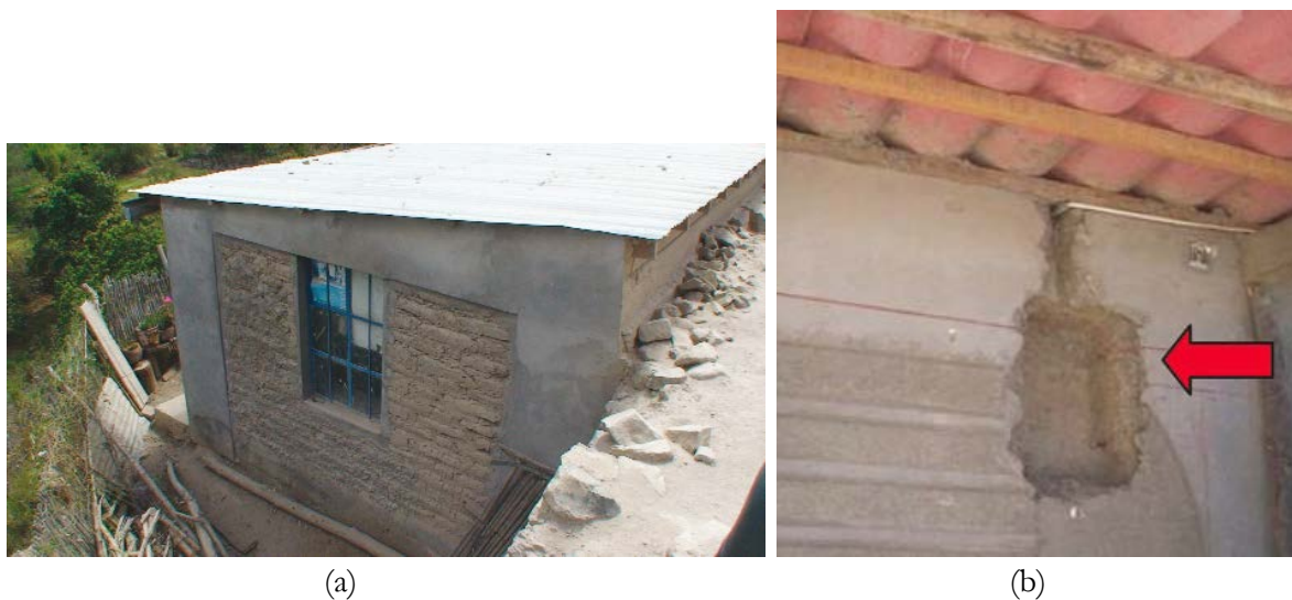
Fig 9. 2001 reconstruction project in Arequipa: Errors in construction or subsequent modifications: a) Rear wall being used as retaining wall to a public road b) Holes cut into wall for electrical and mechanical services, undermining the wall connection and forming a hole in the reinforcing mesh [photo: Chuquimia]
