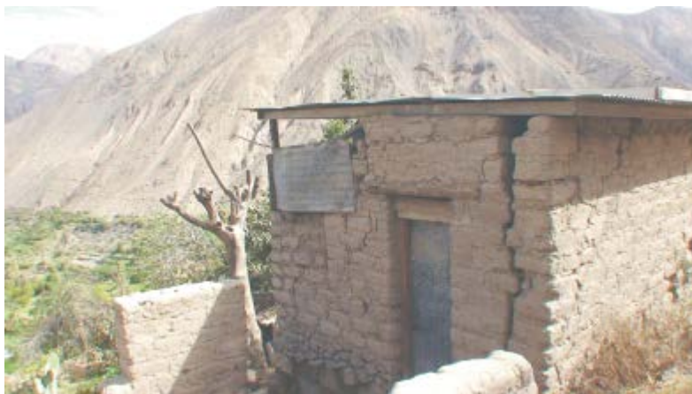
Figure 1. Non-engineered adobe house in Peru showing vertical crack and separation of orthogonal walls owing to out-of plane forces
