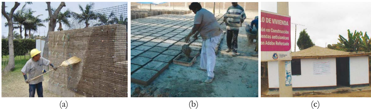
Fig 7. Various stages of the post-2007 reconstruction and capacitation programme: a) Example house reinforced with the plastic mesh, used during the initial training of masons, engineers and NGO personnel (Rubiños) b) Fabrication of adobe blocks in Cañete, carried out by hired masons (Rubiños) c) Completed house in Chinchá Baja, constructed by the public under supervision (after theoretical workshops and practical exercises). Nine houses were completed throughout Cañete, Chinchá and Pisco
