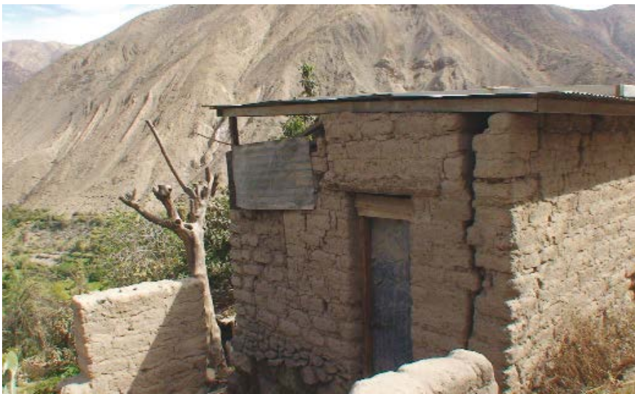
Fig 1. Non-engineered adobe in Condesuyos, Peru. Vertical crack typical of poorly bonded orthogonal walls. Walls are adobe blocks laid in mud mortar. Roof consists of timber planks covered with corrugated sheeting
