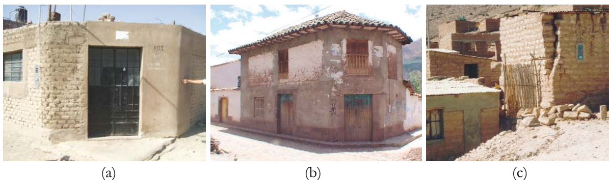
Fig 4. Existing adobe houses retrofitted with steel mesh reinforcement: a) Partially reinforced wall in La Tinguiña. Performed well in the 2001 earthquake b) Two-storey reinforced house in Andahuayllillas, Cuzco c) Reinforced house in Moquegua without damage after 2001 earthquake and neighbouring unreinforced house with severe damage (Quiun)
