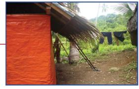
The eaves should extend at least 40 cm past the walls to ensure rain does not get inside.
