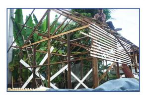
Build frame straight and plumb. Use good quality wood that can be reused in new house. Nail connections firmly and use short pieces of wood to reinforce spliced connections.
