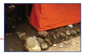
Use rubble to build up a raised platform so the shelter is at least 15 cm above grade. Cover with a layer of screed concrete. Dig a ditch to drain excess water.
