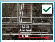
锚固要达0.26m长, 相对弯曲正确。 Anchors should be at least 0.26m long and turned toward each other.
