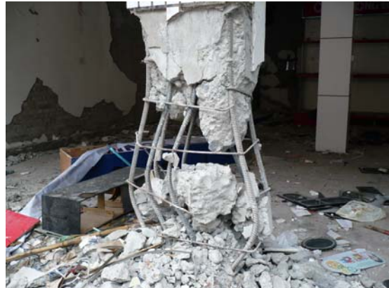
Fig 8. Five story masonry building (6 th column from left in Fig. 7), shear failures in first story columns, note large spacing between ties, lack of hook, and use of large, rounded aggregate, Dujiangyan. IMG0219
