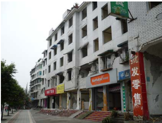
Fig 5. Five story partially confined masonry buildings, damage to open frame ground floor and second floor, Dujiangyan. IMG0183
