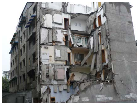
Fig. 2. Partially collapsed six-story unreinforced masonry apartment building with precast concrete plank floors, Dujiangyan.
