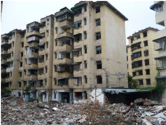
Fig 21. Seven story masonry building with shear cracks, Dujiangyan. IMG0300
