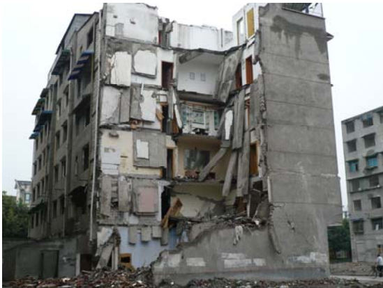
Fig 13. Partial collapse of six story masonry with precast plank floor, Dujiangyan. IMG0267
