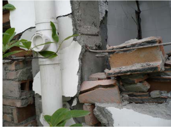
Fig 30. Steel connection between infill wall and column. IMG0668
