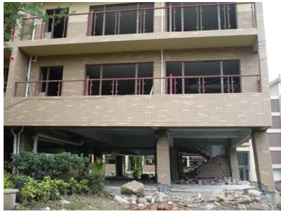
Fig 32. Soft ground story failure of new apartment building IMG0721
