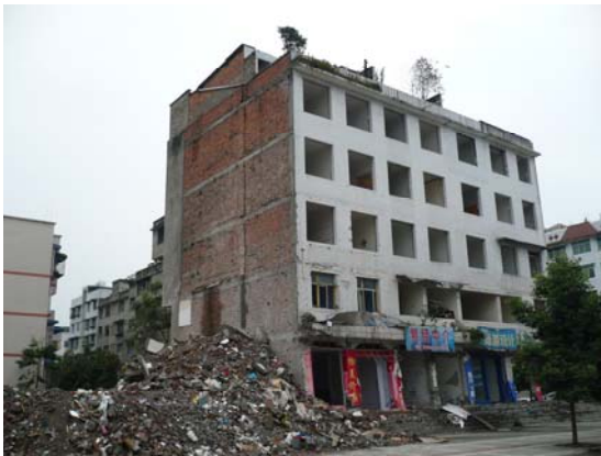
Fig 3. Five story unreinforced masonry building, damage to open frame ground floor, Dujiangyan. IMG0166
