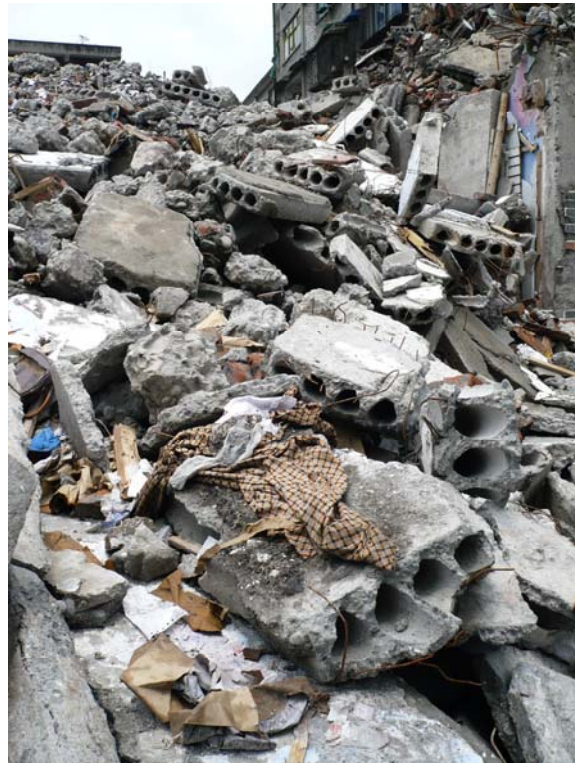
Fig 1. Precast concrete plank rubble, collapsed multi-story unreinforced masonry building, Dujiangyan.
