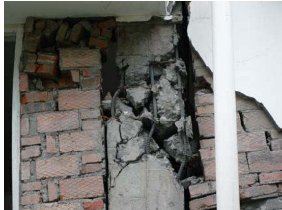
Fig 24. Shear failure at top of ground floor column, six story building from Fig. 23. IMG0705
