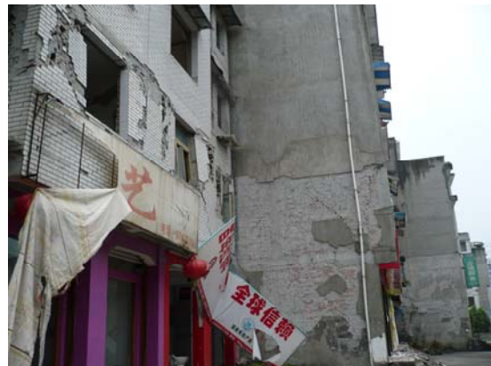
Fig 6. Five story partially confined masonry buildings (Fig. 5), damage to open frame ground floor and second floor, Dujiangyan. IMG0189
