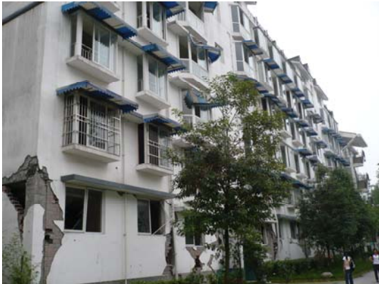
Fig 23. Damaged six-story reinforced concrete frame with masonry infill, Dujiangyan. IMG0714
