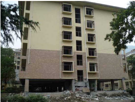
Fig 31. Damage to ground floor columns, new six-story apartment building, Dujiangyan. IMG0718
