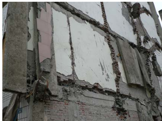
Fig 12. Side view of five story building (Fig. 10), note lack of connection between ground story column and upper floor columns and beam. IMG0254
