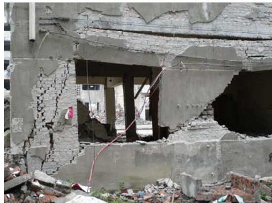
Fig 18. Shear failure in ground floor masonry, building shown in Fig. 17 (left) and Fig. 10. IMG0266
