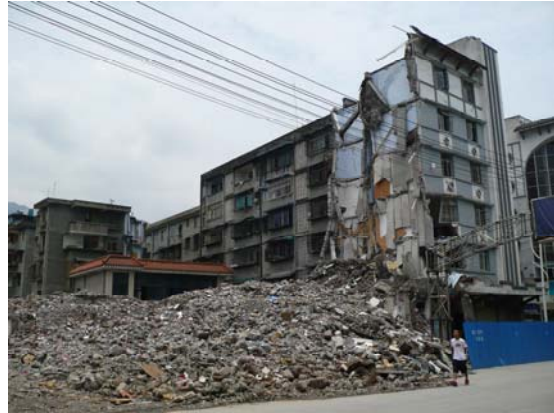
Fig 20. Partially collapsed URM with precast concrete plank, Dujiangyan. IMG0335
