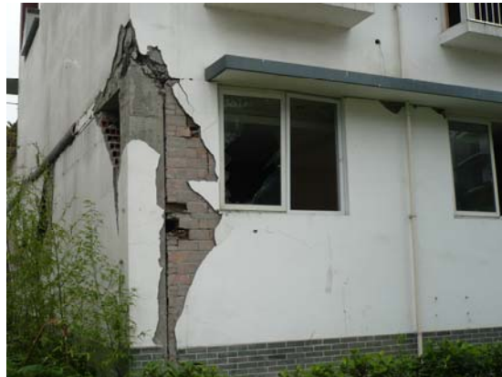
Fig 26. Shear failure in corner column. IMG0712
