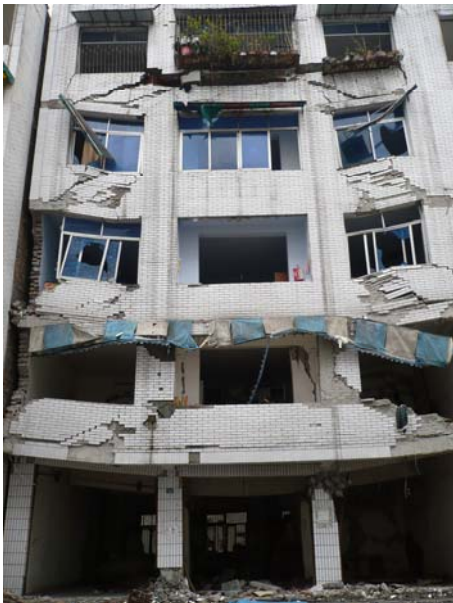
Fig 9. Five story masonry building, collapse probably prevented by adjacent buildings, Dujiangyan. IMG0243
