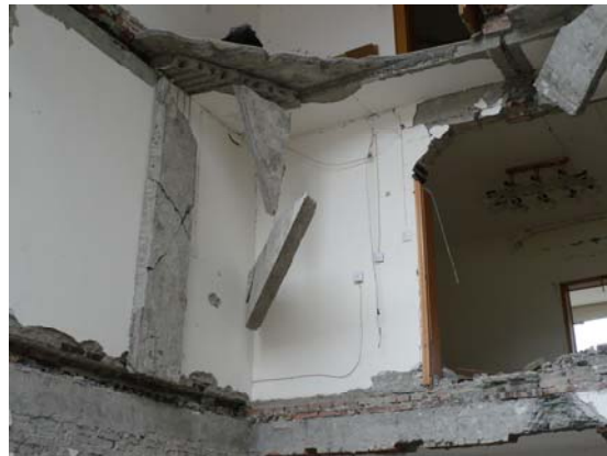
Fig 16. Close-up view of partial collapse of building in back of Fig. 15, note precast planks resting on top of, rather than connected to, ring beam, Dujiangyan. IMG0280
