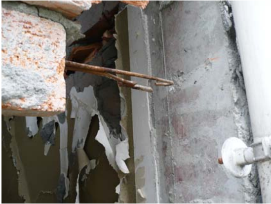
Fig 29. Steel for connection between infill wall and column, note that bolt holes in column have been plastered over. IMG0711
