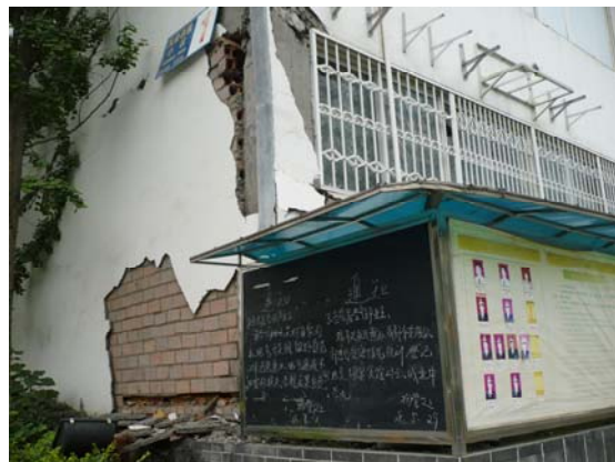
Fig 28. Overturning failure of masonry infill wall. Shear failure in corner column. IMG0717
