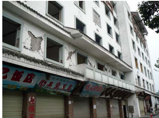
Fig 22. Shear cracks through columns in six-story confined masonry building, Dujiangyan. IMG0307
