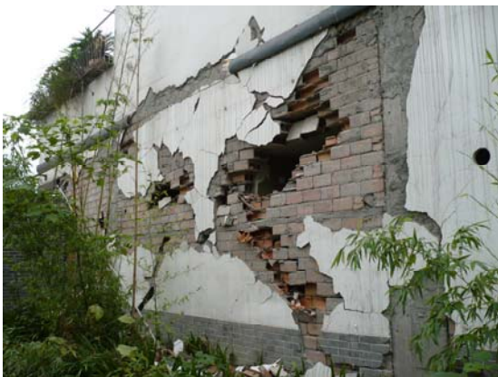
Fig 27. In-plane shear failure of masonry infill wall, note that thin horizontal band at mid-height was not sufficient to prevent crack propagation. IMG0715
