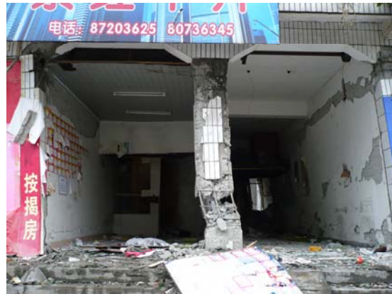
Fig 4. Five story unreinforced masonry building (4 th column from left in Fig. 3), shear failures in first story columns, Dujiangyan. IMG0168
