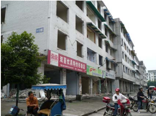
Fig 7. Five story masonry buildings, damage to open frame ground floor and second floor, Dujiangyan. IMG0216
