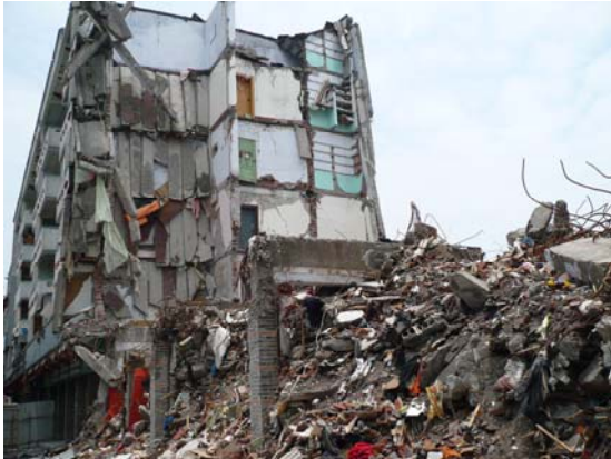
Fig 19. Partially collapsed URM with precast concrete plank, Dujiangyan. IMG0324
