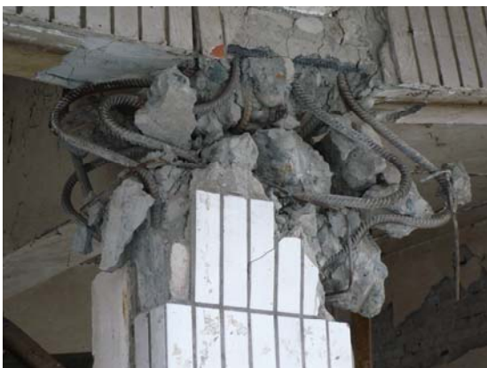
Fig 11. Ground floor column failure (rightmost column in Fig. 9), Dujiangyan. IMG0240
