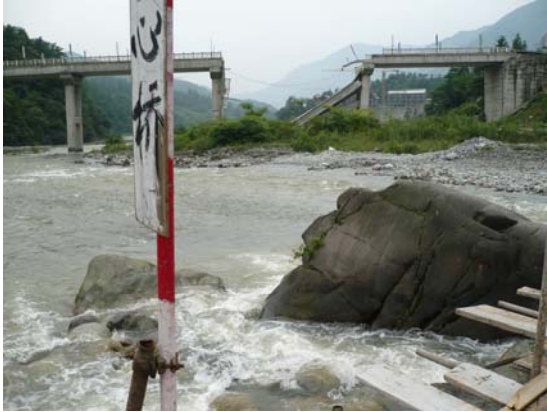
Fig 9. Gao Yuan bridge looking west from temporary footbridge. IMG0458
