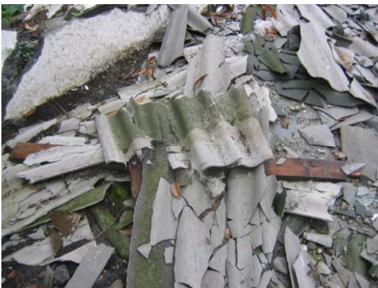
Fig 11. Corrugated cement and fiber sheets. IMG1130
