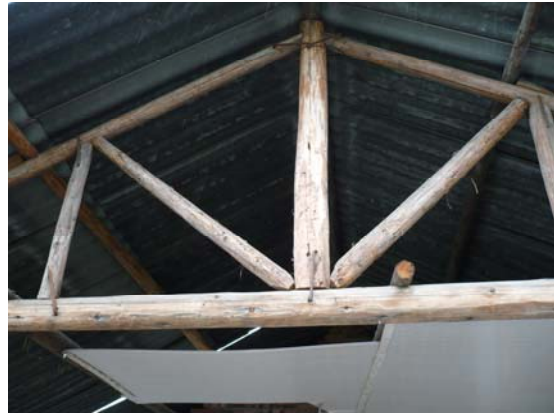
Fig 10. Typical truss. IMG0098
