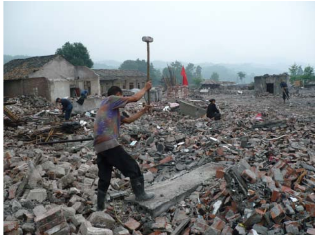
Fig 1. Debris removal and recycling in heavily damaged Danan Village. A few unreinforced masonry buildings with timber roofs remain standing. Collapse of unreinforced masonry buildings with precast concrete roof/floor planks (shown under the worker's right foot) contributed to the majority of casualties in both urban and rural areas visited during the reconnaissance.
