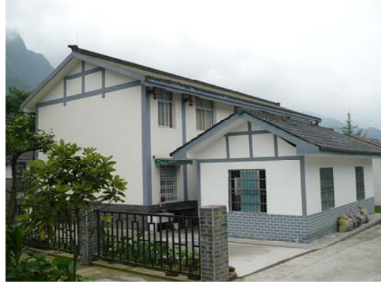
Fig 14. Single story URM with timber roof, no damage (two story building is confined masonry, described later), Gao Yuan village. IMG0560
