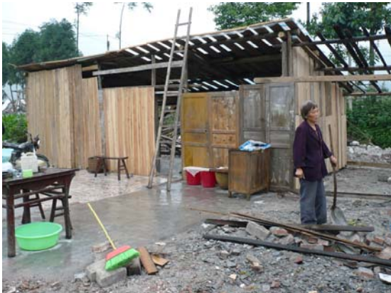
Fig 29. Homeowner-built transitional shelter, rural Pengzhou. IMG0072
