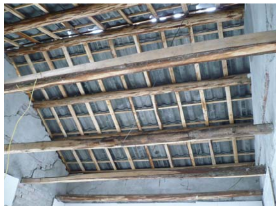
Fig 18. Use of more modern roofing tiles with ridges to prevent displacement. IMG0031
