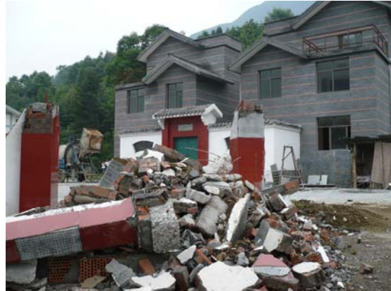
Fig 24. Two-story confined masonry, no damage, tiled exterior, collapsed URM gate in foreground, Gao Yuan village. IMG0545
