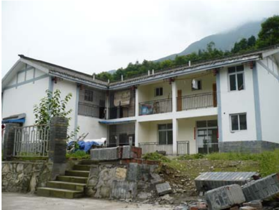
Fig 23. Two-story confined masonry, no damage, Gao Yuan village. IMG0552
