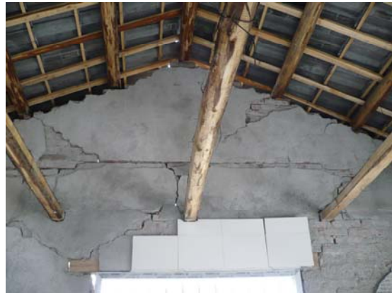
Fig 16. Interior unfinished gable wall, Gao Yuan Village. IMG0573
