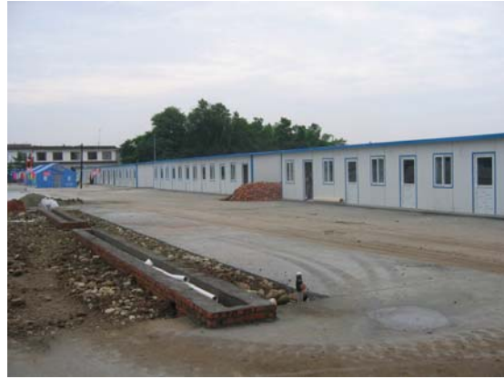
Fig 28. Transitional shelter near Jiezi. IMG1163
