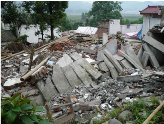
Fig 19. Collapsed URM with precast concrete plank, near Xiao Yu Dong Bridge. IMG0433
