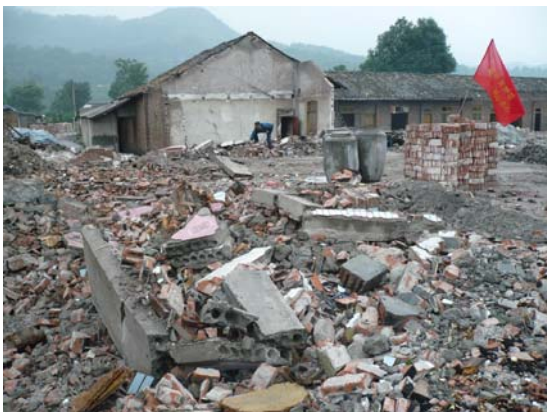
Fig 5. Partially collapsed unreinforced masonry with timber roofs in background, collapsed URM with concrete plank in foreground. Rural Pengzhou. IMG0122
