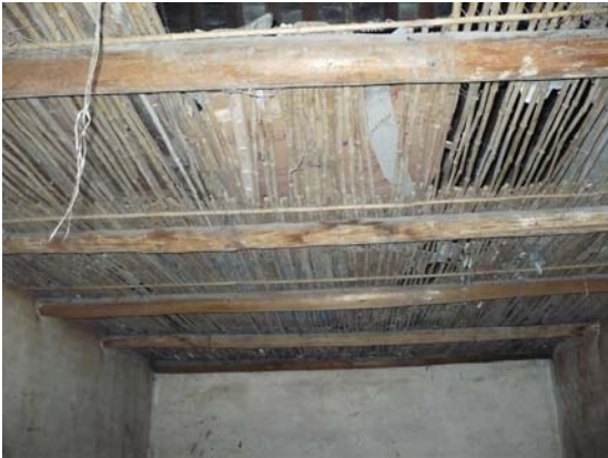
Fig 9. Typical ceiling. IMG0115
