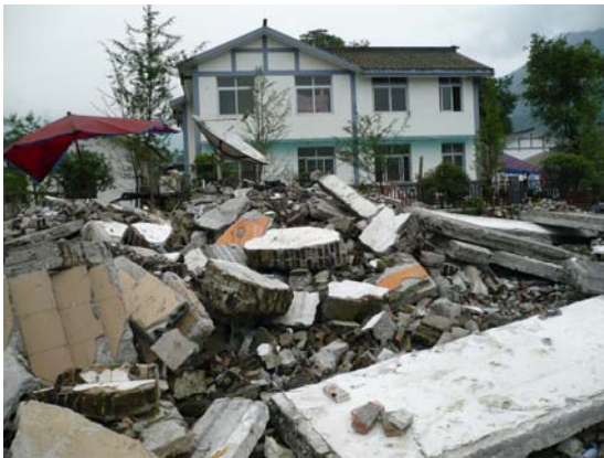
Fig 25. Two-story confined masonry, no damage, collapsed URM with precast plank in foreground, Gao Yuan village. IMG0586
