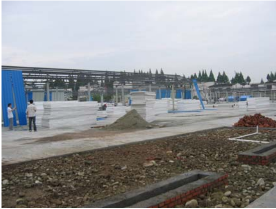
Fig 27. Transitional shelter near Jiezi. IMG1164
