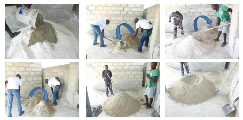
Shifting the pile from side to side at least three times will help ensure the UNIFORM COLOR of the mix.
