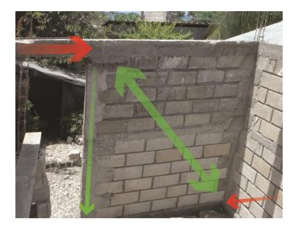
In many badly designed REINFORCED CONCRETE structures, the walls still carry much of the seismic load so the quality of the blocks used remains extremely important.
